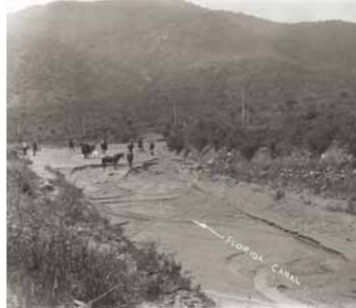
Embanque Canal Florida 1915
